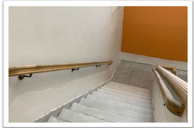
Walls are being patched and painted in stairway three.
