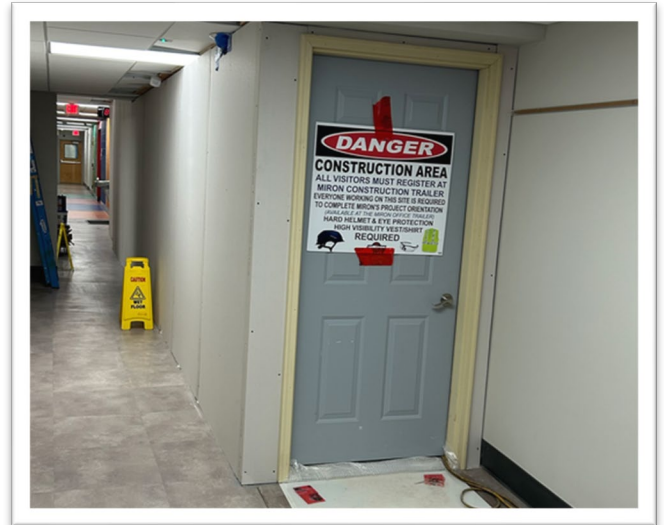
Temporary partition around the gym bathrooms.
