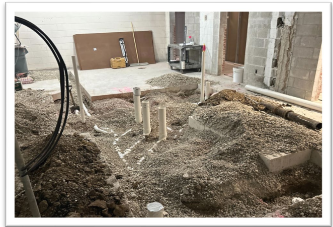
Underground plumbing rough-ins for the gym bathrooms.
