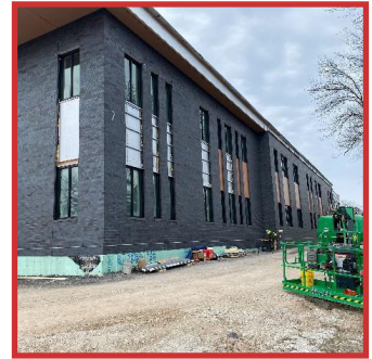
Exterior metal panels are being installed.
