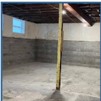
Locker room demolition has been completed.
