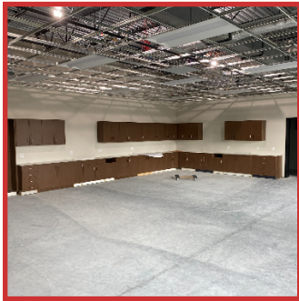
Cabinets and other woodwork have been added to lab classrooms.
