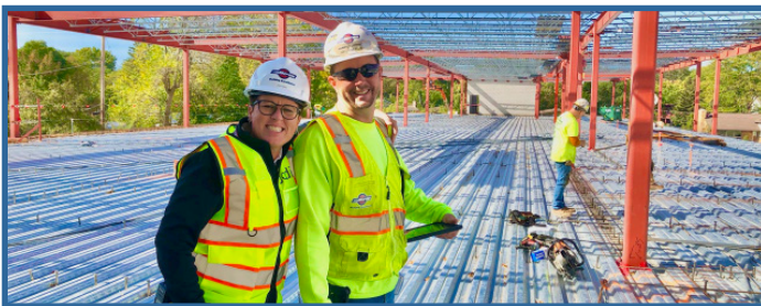
Principal Jodi Hackl visiting the Bayside construction site.
